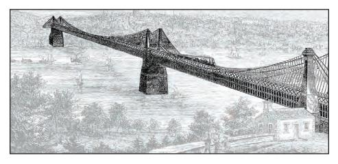
The original design of the Poughkeepsie Railroad Bridge in the 1870s shows a suspension style construction similar to the Brooklyn Bridge that was never realized. This image looks from the west bank of the Hudson toward Poughkeepsie. Where: The
